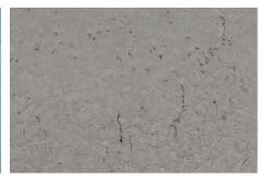
Small, fine cracks on the surface of concrete are very common within the life long curing process and do not impact the structural quality or performance of the basin. If you are concerned about the placement or size of any cracks please do get in touch.
