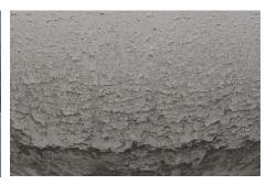
The liquid state of concrete when it is being cast means that textural flow lines can sometimes be visible on the surface of the concrete. This tends to be more visible when casting curved or tall vertical surfaces and is another typical characteristic of concrete.
