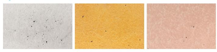
Due to the nature of the casting process, air trapped within the concrete can sometimes cause small holes to form within the surface. These can vary in size and add to the distinctive texture and aesthetic of concrete.
