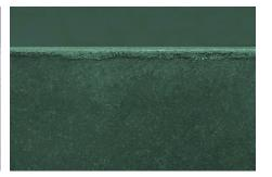
Some basins require two-part moulds which can result in a different texture around the edge where the two moulds meet. This is where moisture within the mix can evaporate out at the seam creating a more raw, distinguished texture.
