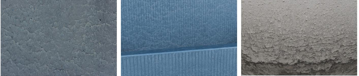
The liquid state of concrete when it is being cast means that textural flow lines can sometimes be visible on the surface of the concrete. This tends to be more visible when casting curved or tall vertical surfaces and is another typical characteristic of concrete.
